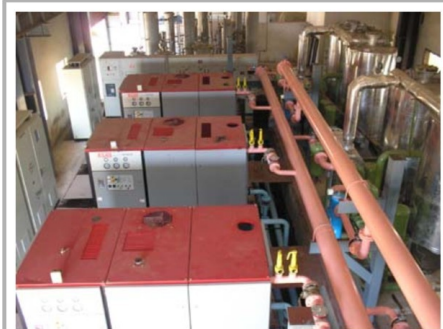
ELGI oil-free compressors at an installation
