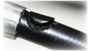
Real life problem 3 Damaged Pneumatic Tools
