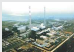
Thermal Power Projects
